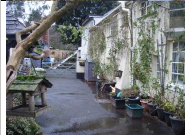
Flow followed down path down to garage at rear of The Mews, SX9150370569 looking NW
