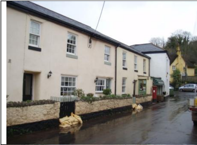
View of sandbagged properties (1&2 Orchard Cottages – gardens flooded) towards Post Office. SX9158970520 looking W
