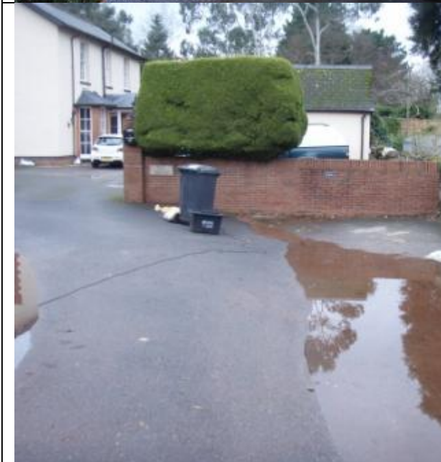
Low point showing remaining water on driveway to The Gables, SX9149870564 looking NW
