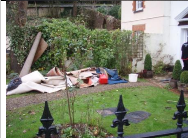
Flood damaged property at the Gables SX9147570568 looking W
