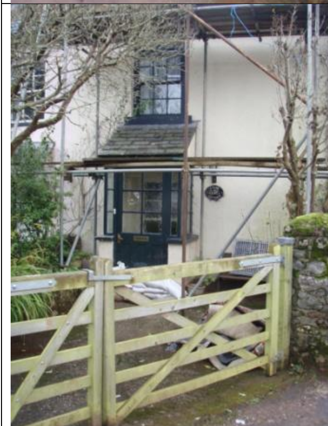
Damaged carpets outside Lilac Cottage, SX9150570551, looking SW
