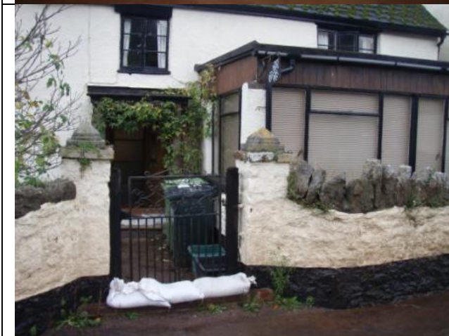
Old Bailey Farm – resident managed to keep flood water out of property through combination of raised steps and sandbags. He complained that vehicles driving through the village were creating bow waves which overtopped his defences by the gate. SX9158270528 looking NE
