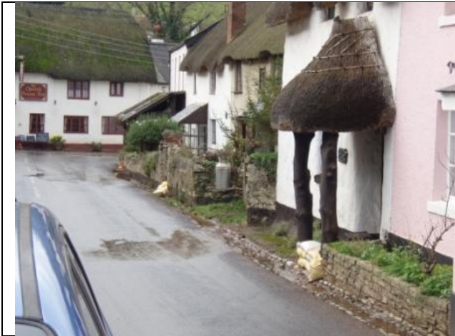
Sand bagged properties on Deane Road SX9164570516 looking W
