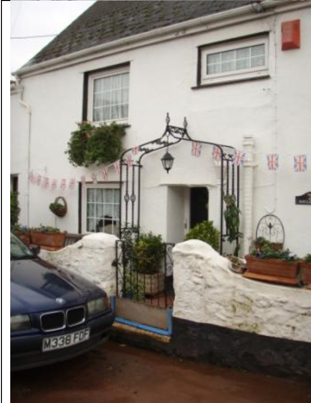
Daylesford, improvised flood board on gate – not reported flooded. SX9157170539 looking NE
