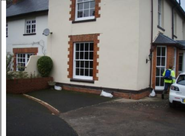
The Gables, sandbags over airbricks SX9148070570 looking NW
