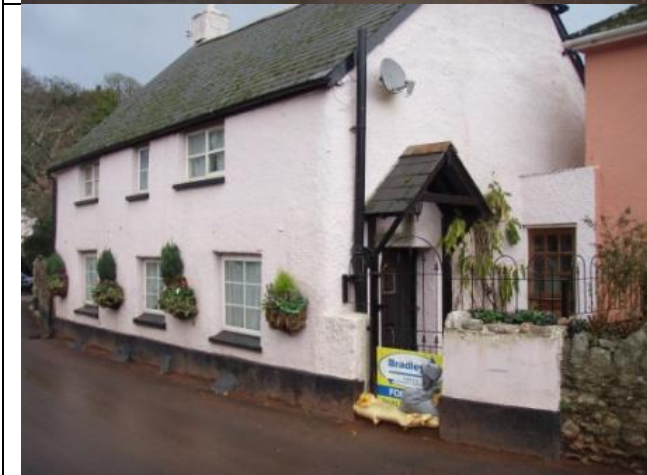
Rose Cottage, uphill door sandbagged, SX9162970467 looking NE
