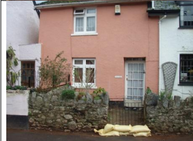
School house sandbagged and flood boards on front door – not reported to have flooded, SX9162970467 looking E
